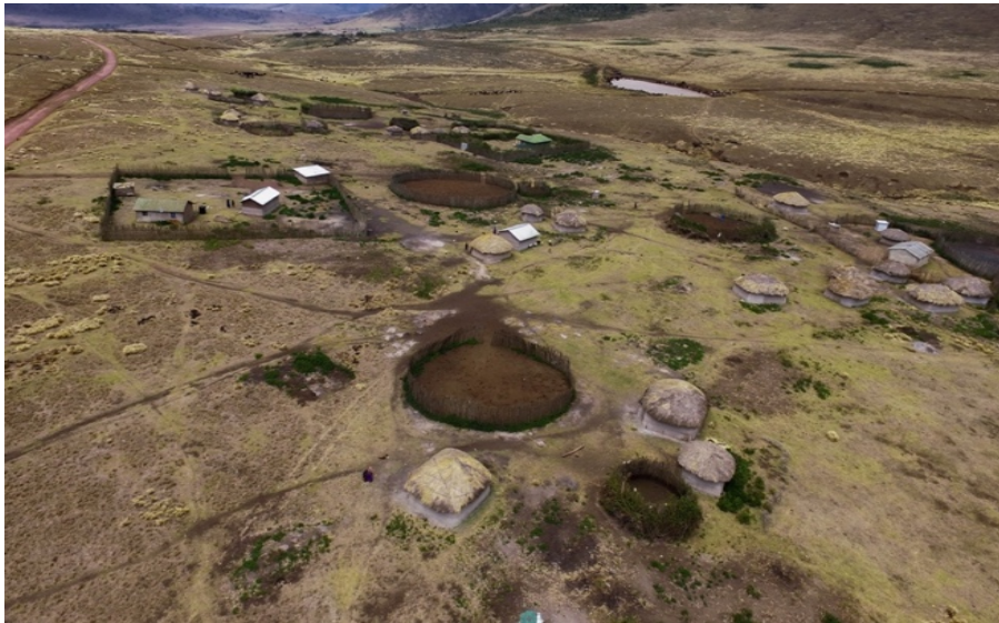
Fig. 1. A Maasai homestead undergoing a transformation: note fragmentation of the homestead, fences on exotic houses and horizontal sprawl. Source: fieldwork 2019.
