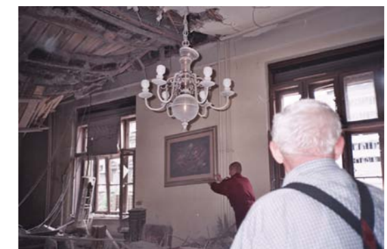
Figure 5. Condition of the building during the salvage.
