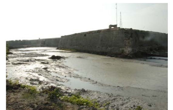
Figure 6. Rampart and the moat after conservation, Dutch Fort of Jaffna.
