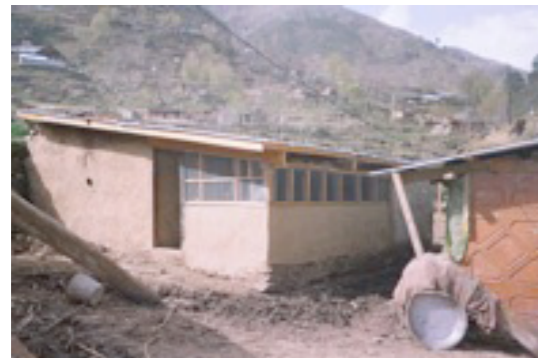
Figure 4. Kodar village. Shelter reconstructed with local materials.
