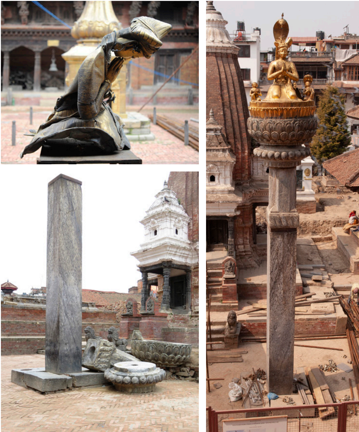
▲ Fig. 28. The Pillar of Yoganarendra Malla after the earthquake (left) and after its successful conservation and re-erection (right) (Institute of Conservation, University of Applied Arts Vienna, 2015-2017)
