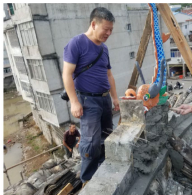
▲ Fig. 26. Ji Haibo documenting the restoration process
